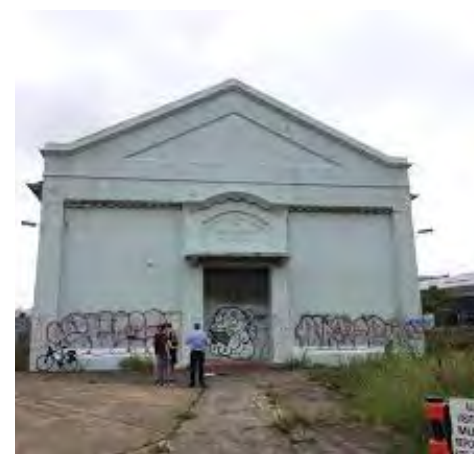
Sydney Water Valve House
