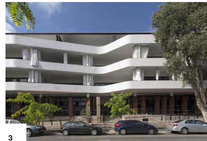
3 Casba, Danks Street
